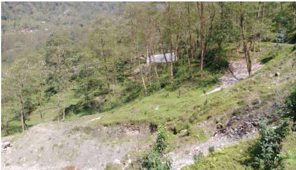
Fig 15: Showing slided scar in slope wash material below road to school.
