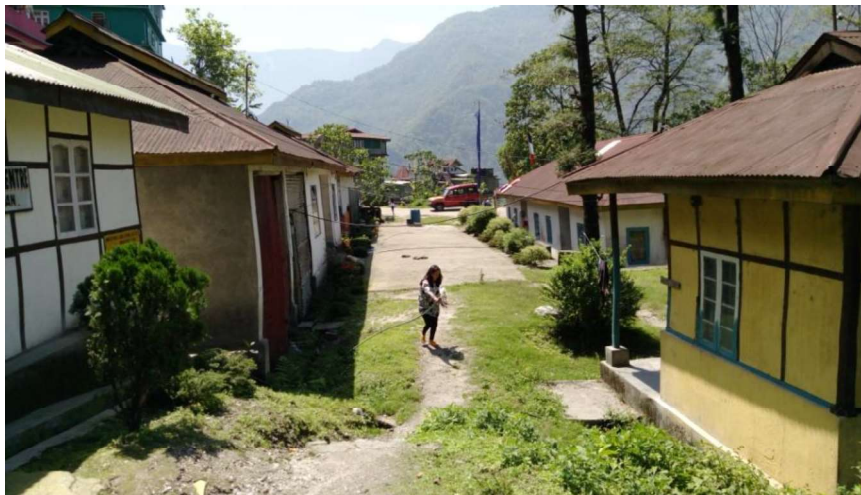
Fig 5: Showing old Mangan Bazar left side of the slide zone below SNT complex.
