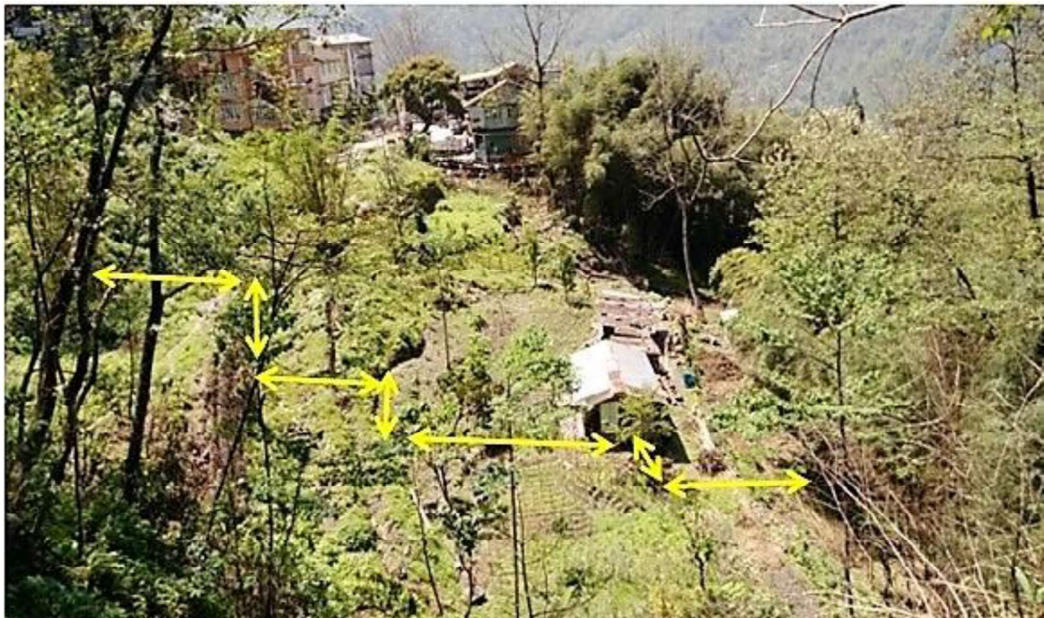
Fig 11: Showing steps due to sequential subsidence in the slide mass below SNT complex
