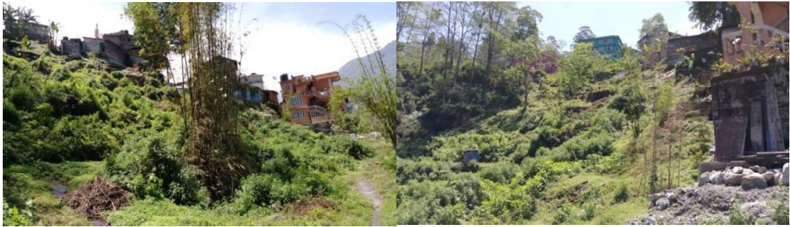
Fig 8: Showing right & left portion of the crown of slide zone below SNT complex
