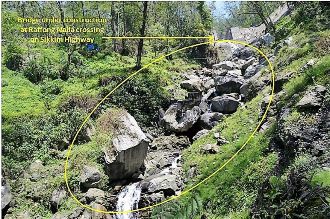
Fig 18: Upstream view of Raffong Nalla showing accumulation of huge boulder along Nalla below Sikkim highway.
